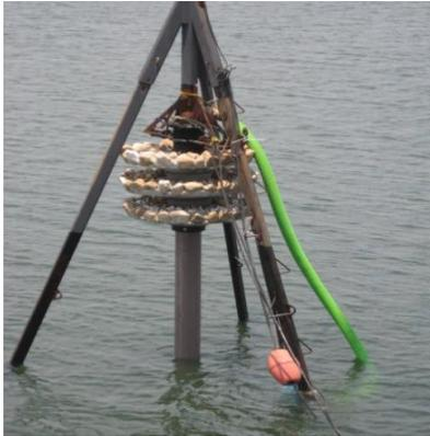
The reefs consist of multiple piling-mounted Eco Systems made in Gulf Shores, AL. Materials are thin concrete discs covered in Florida limestone rock and mounted on environmentally friendly composite pilings which are driven into the seabed. Three to four discs each 5ft in diameter are mounted on each piling and the individual reef structures are placed 10 - 20ft apart.
